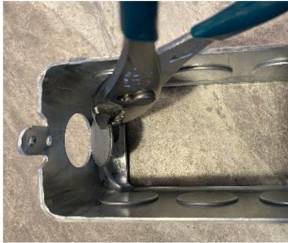
Figure 17: A pair of pliers is used to remove the metal hole covers from the box as detailed in step 1 of this procedure.
