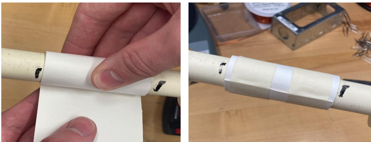
Figure 20: The strip of paper is wrapped around the PVC pipe and taped in the manner described in step 4 of this procedure.
